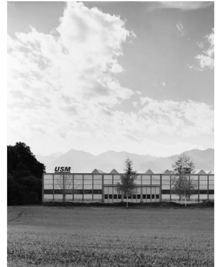
Founded in 1885 and headquartered in Münsingen, Switzerland, USM today is still a family-owned and family-led business, now in its fourth generation.
